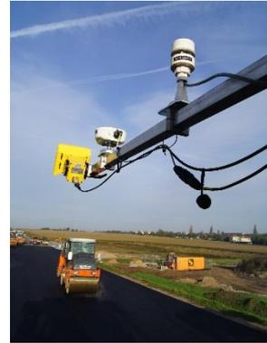
*The scanner scans the asphalt temperature for the whole project*
