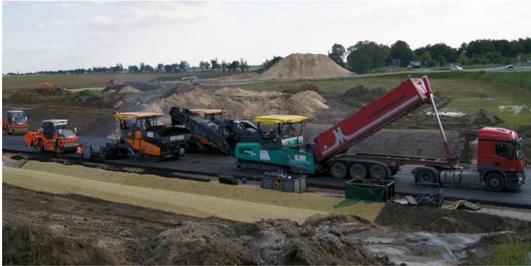
*Two PAVE-IR Scan systems were used during the new construction of the B6n bypass in Germany.*
